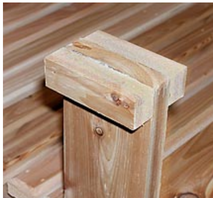
Attach cleats to both sides of each front upright.
